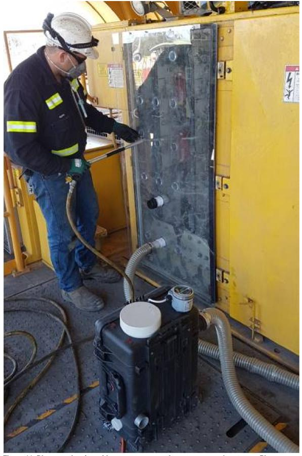
Figure 11. Blow-out cleaning with a prototype containment cover and prototype Plev
