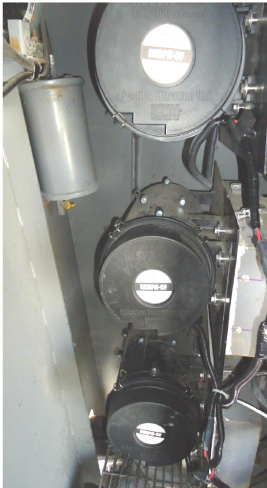
Fresh Air Intake Three RESPA-CF Units
