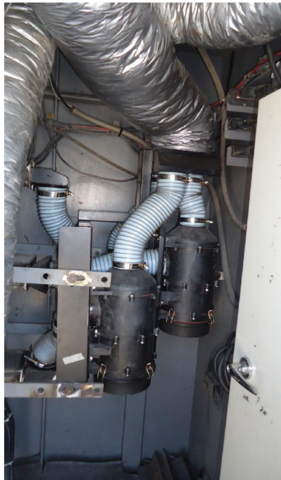
Recirculation Air Three RESPA-FFX Units
